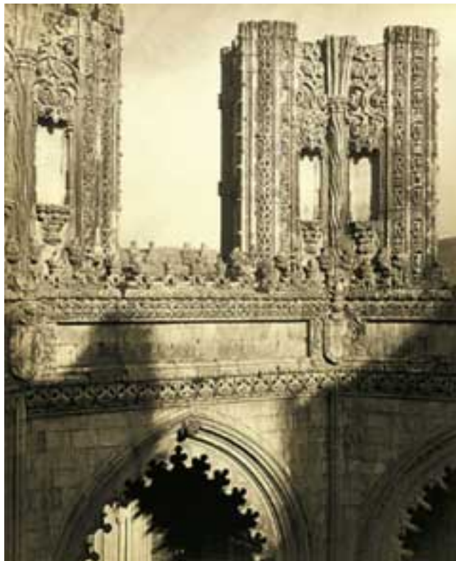
Monastery of Batalha. Capilla Imperfeita; view of towers above archway, from the North 38,75 x 31,5 cm. (V&A 58371)
